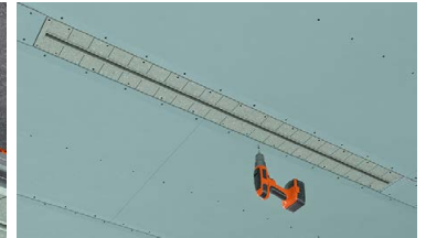
Important: During installation, all fixing screws must be fully tightened.
